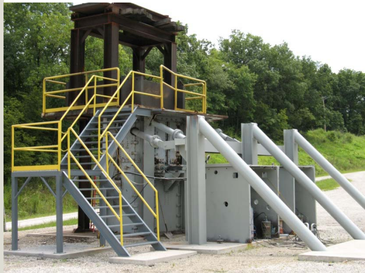
Vertical Test Fire Stand
